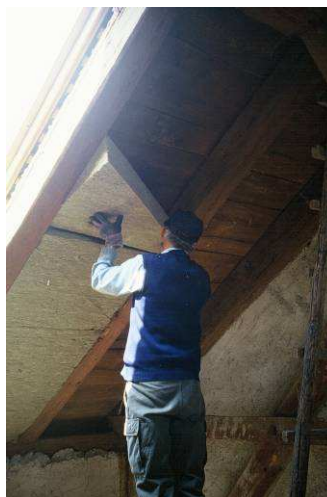
Figure 12: Insulation of the roof layer (M.Tomšič)
