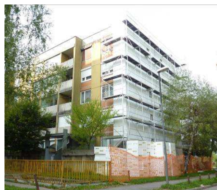
Figure 7: Thermal renovation of an existing building (M. Skubic)
