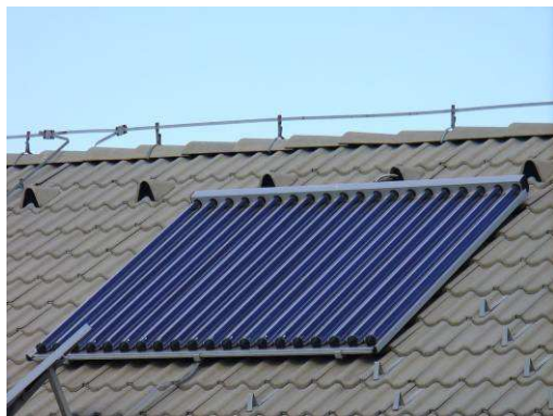
Figure 20: Solar collector (M. Skubic)
